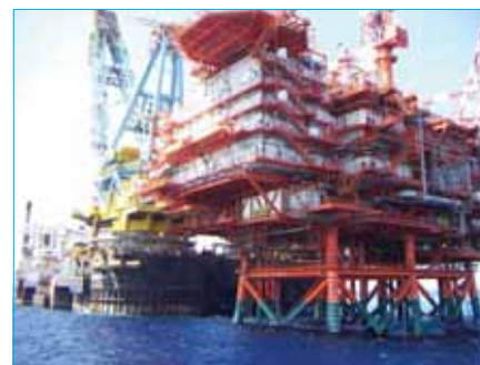
The Sabratha platform, (above) and a view of some of Weatherford's plant for precommissioning (below).
