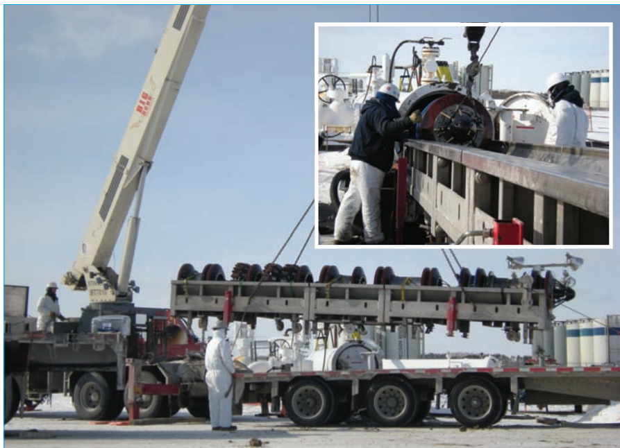
GE's tool arriving and (inset) being prepared for launch, on the Keystone pipeline inspection project.
