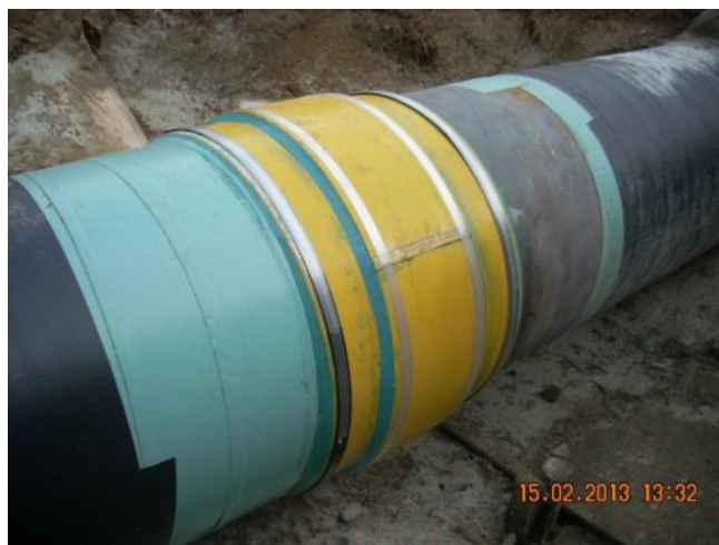
Clock Spring apply metal marker bands to composite sleeve
