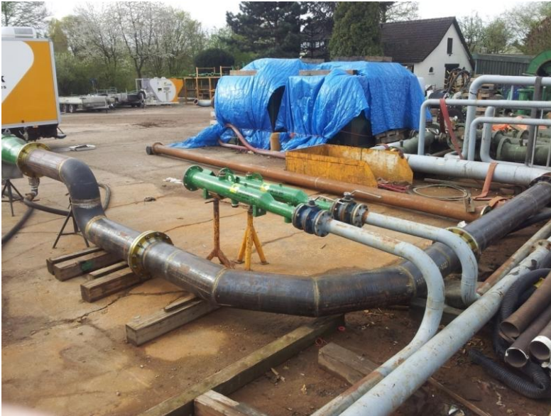
Figure 4: Mock-up to prove piggability of the new developed Piglet inspection tool
