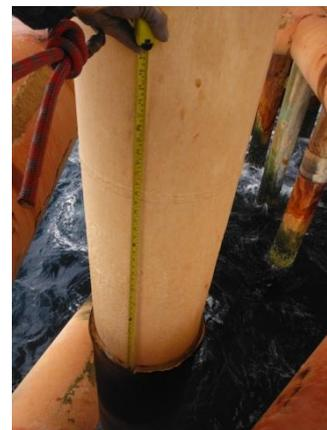
Figure 6: Locating External Corrosion on the Captain Oil Export Riser
