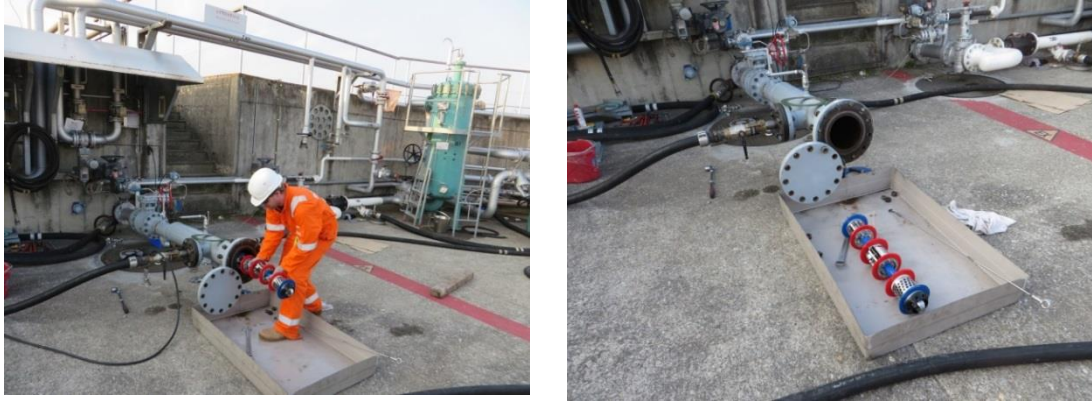
Figure 2: Launching (left) and receiving (right) the tool
