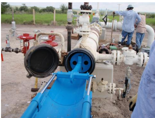
At site: launcher fully loaded with 6 AMPL pigs
