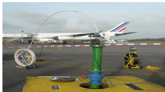
Push Pull system inspecting an airport hydrant system
