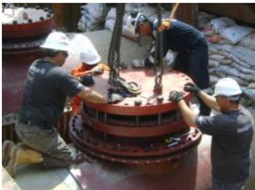
Installation of blind flange on the gland fitting for hydro testing
