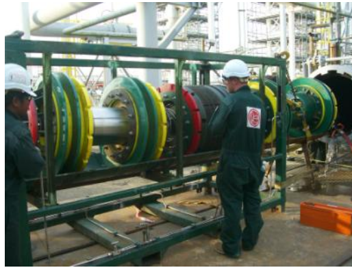
STATS isolation technician Iain Reid, prepares 36" Remote Tecno Plug™ for deployment
