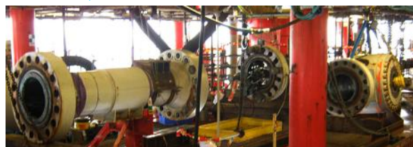
ESDV being rigged out
