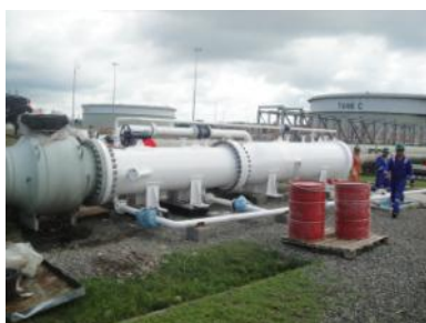
Serck Services' Pig Launcher Receiver
