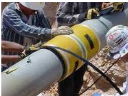
Figure 2. Clock Spring Marker Bands being installed
