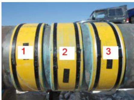
Figure 3. Clock Spring Marker Bands installed as per standard procedure
