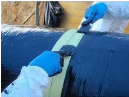
3X Engineering's composite repair
