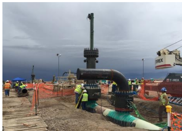
STATS Group Cortez 24 inch bypass line installation
