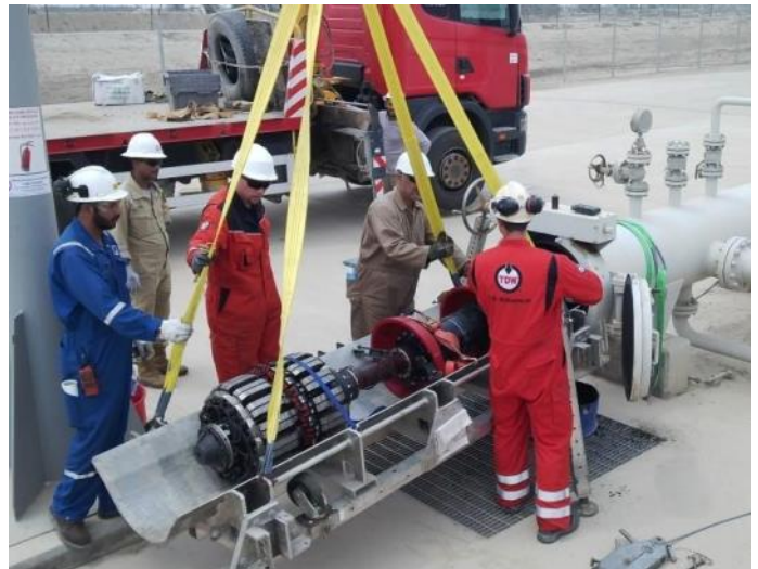
T.D. Williamson uses KALIPER® 360 tool and gas magnetic flux leakage technology to prove pipeline integrity
