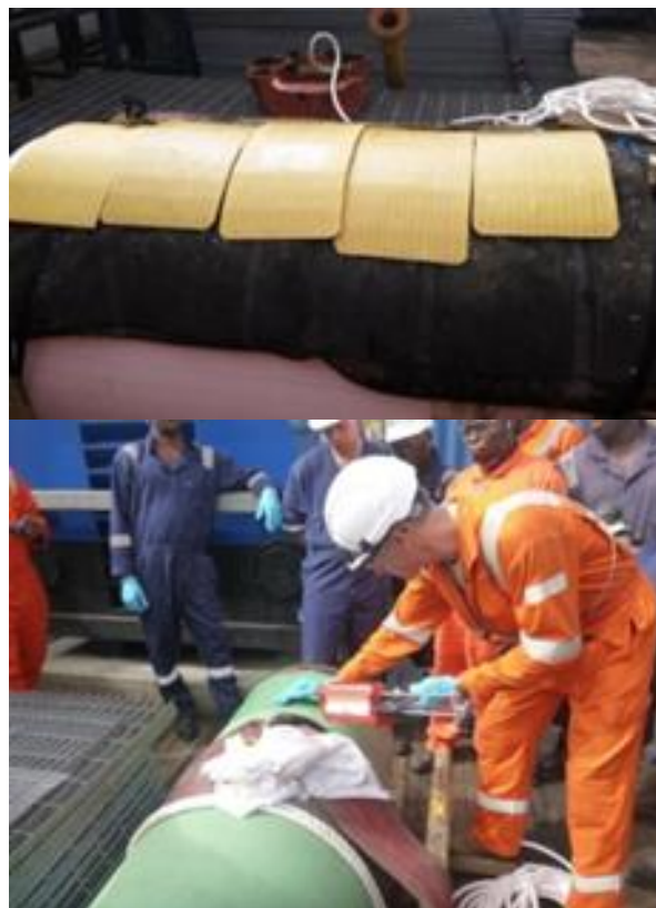
Composite plate manufacture on the foot print of the dented area & primer application (training picture). ●
