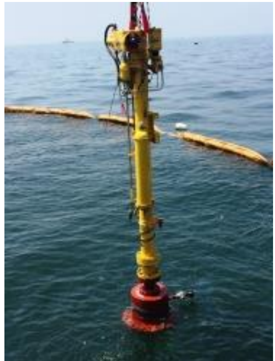
First subsea application of STOPPLE isolation technology in Japan.
