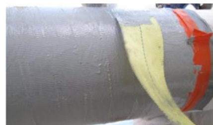
Wrapping in progress ●
