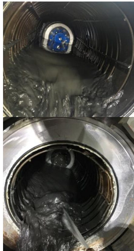
Pipeline Cleaning at worksite
