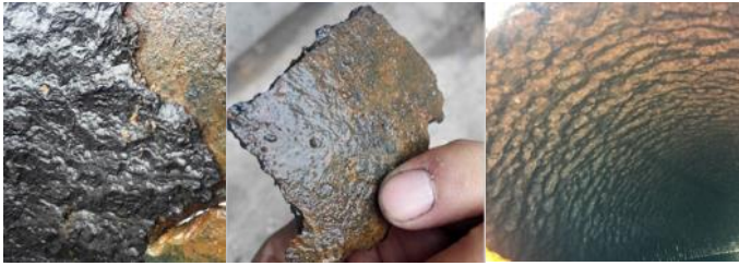
Internal views of the pipeline before cleaning
