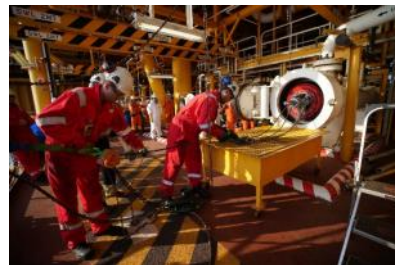
Pig successfully recover to the launcher
