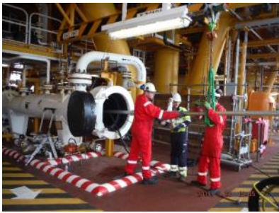
Deployment for pig recovery tool
