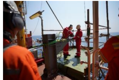
Wire attached to hydraulic cylinder and strong hold behind the launcher
