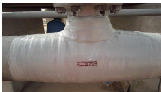
Wrapping completed (12 layers) & ID plate installed ●
