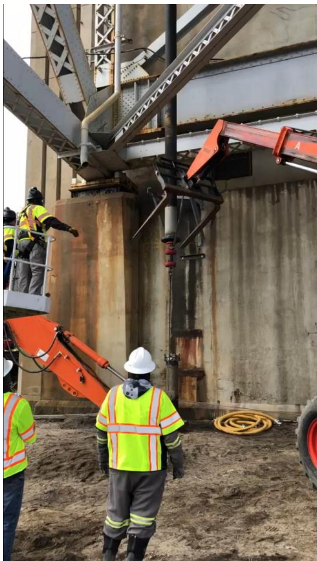
ILI tool being removed from the pipe
