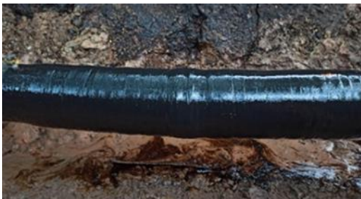
View of the repair completed
