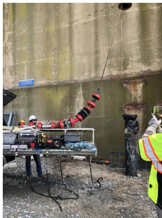
ILI tool being inserted into the pipe
