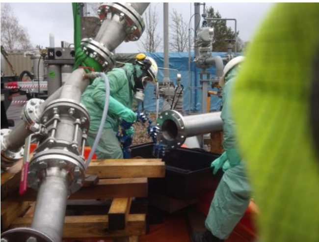
Removal of mechanical cleaning tool (MCT)
