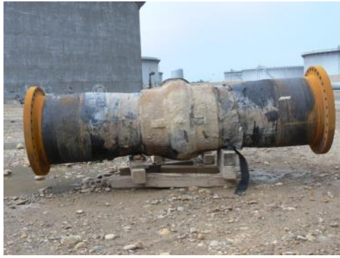
06:00 view of 30" gate valve removed from the line
