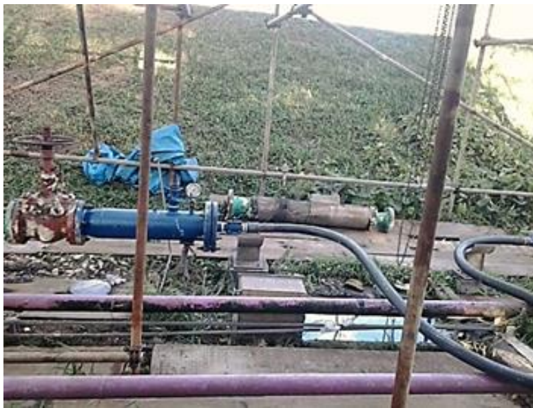
Station pig launching station
