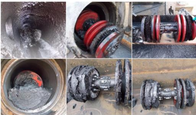
Pig runs in 10 inch gas export pipeline
