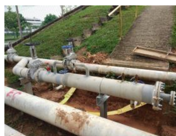
Custom-built lateral WYE launchers and receivers were installed allowing for inspection without disrupting product flow.
