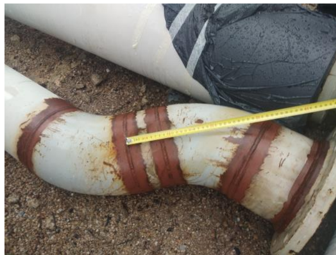
Challenging pipeline features are replicated and tested at Dexon's 6 acre on-site test yard as part of Dexon's inspection verification program.
