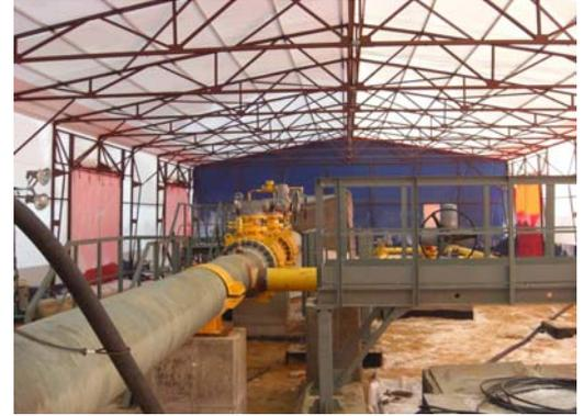
Figure 13: Above ground pipeline section protected by habitat
