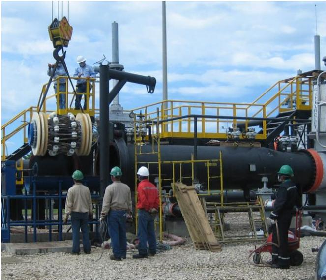
Fig. 4: GEO inspection tool being installed into the trap
