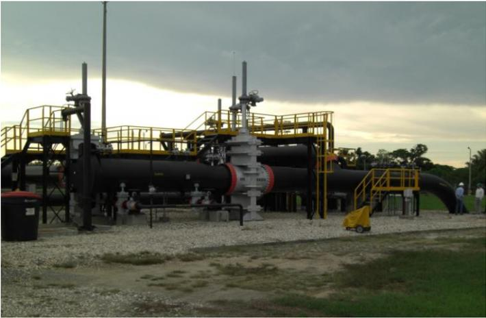
Fig. 2: Pig trap at Ocesa's terminal, Covenas, Colombia
