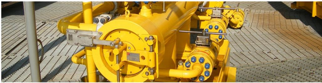
The locking system prevents the operator from operating a valve when it is not allowed and the valve can only be operated with the designated key. Each lock is operated by two keys, one released in the open position and one in the closed position. By using unique keys that travel between locks the key codes can be designed to guarantee the steps of operation and guide the operator through the sequence.
