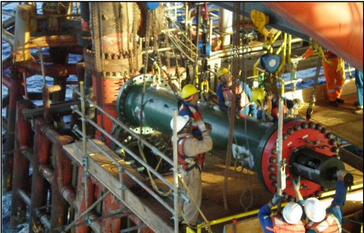
**Figure 13: 30" BISEP™ Launcher Rigged into Position**
