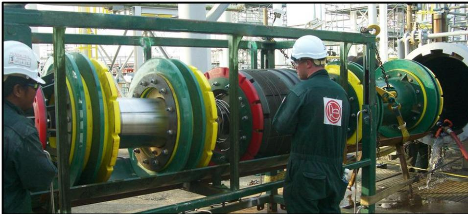
**Fig 8: 38" Tecno Plug™ Deployment Malaysia**
