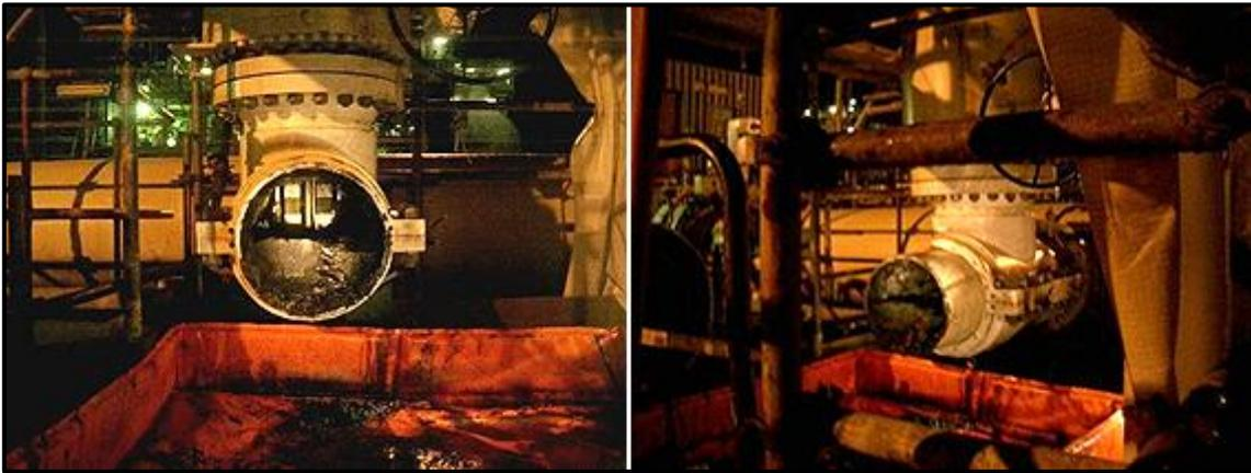
**Figure 11: BISEP™ Isolating Pipeline On-Site with Dead Leg Cut Away**
