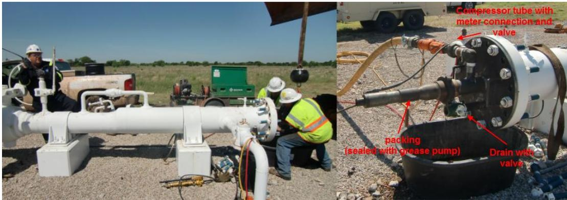
Figure 13: Tool loading (left) / launcher set-up (right)
