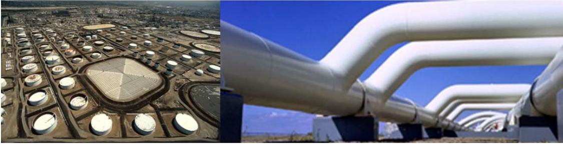
Figure 7: Branch connections inside a tank farm (left) / gathering lines (right)
