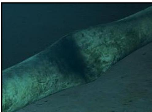
**Figure 1: Unpiggable Defect in Pipeline**
