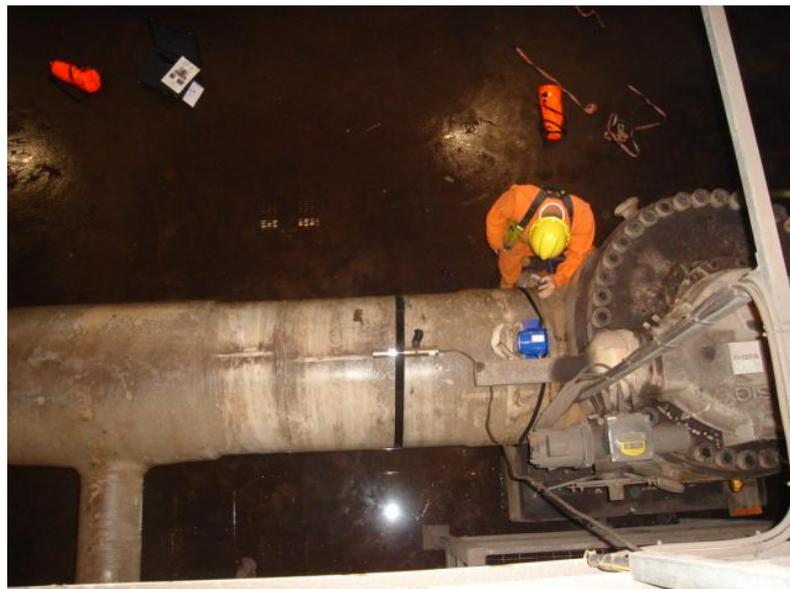
**Pipeline in pit at beach valve station with 3003X antenna strapped to the pipe wall. A cable connected to the antenna transmits signals received to the 3002X Receiver at the pit's surface.**
