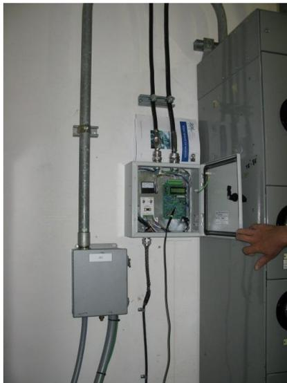
**3002E Receiver mounted at remote valve station monitoring cabin**
