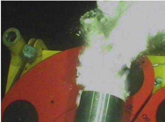
Once cured, the EVO-Pig LG dewatering train was then successfully pushed through the riser and pipeline using nitrogen as the driving medium.
