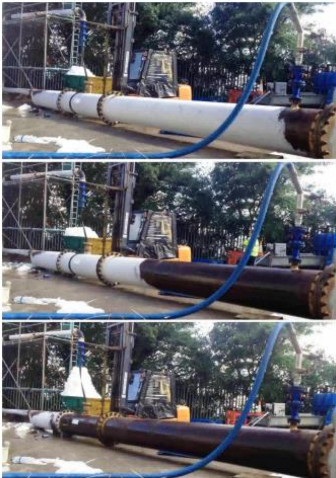
Figure 3 Ice pigging was performed on a dual diameter 24" to 8" steel pipe. The ice and push-water were inserted through a 2 ½" hose connected to a 2" inlet. Frozen condensation on the pipe shows the progress of the ice plug through the constriction.
