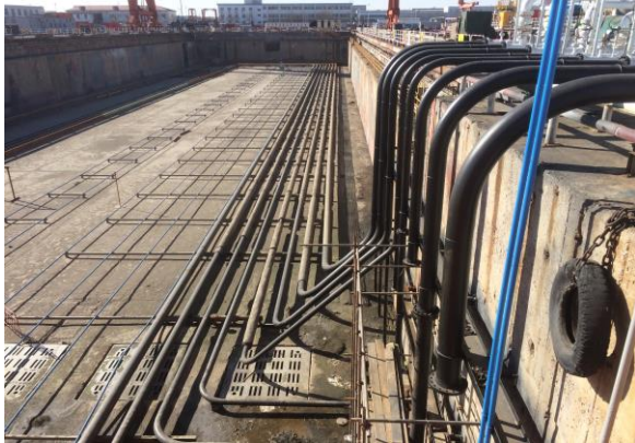
Figure 3: Operator's test loop located in a dry-dock.
