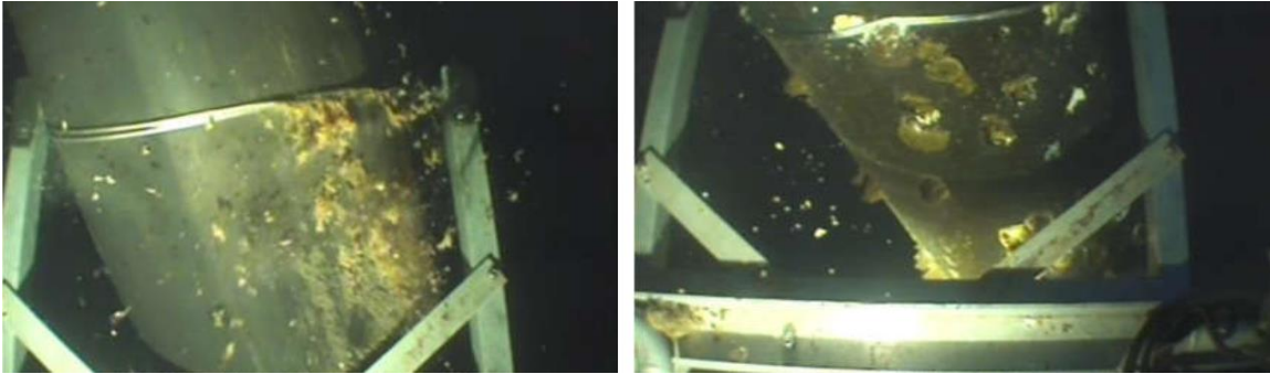
Figure 3: Marine growth removal utilizing the “cheese wire” tool
